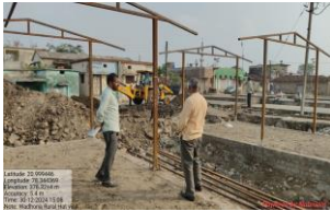
Construction work of Rural Haats
