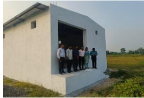
Construction of shed for the turmeric boiler plant
